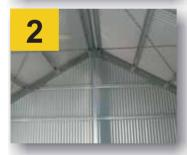
Tilmac galvanised purlin frames are strong with the option to choose from heavy duty C150 to C300 purlin frame.
