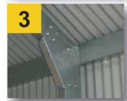
Fully bolted connections are made from galvanised steel for added strength and protection. The bolts guarantee secure fastenings down in all weather conditions.
